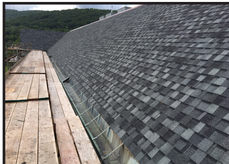
The Port Dickinson roof shingles have been replaced.
