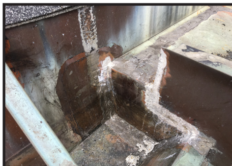
Repair work to the copper gutter at Port Dickinson is complete.
